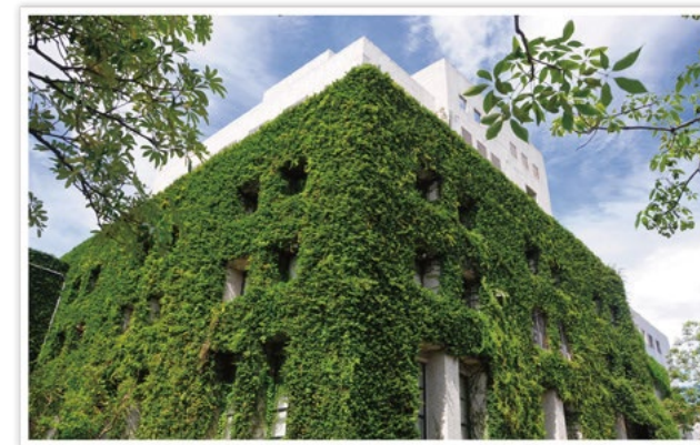
Green planting on the outer wall of the library
